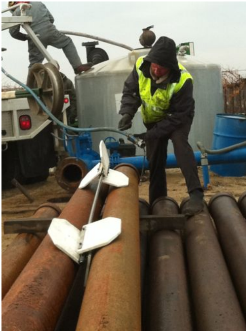
Preparing the centralizers – adaptable for ID 2" – 48"
